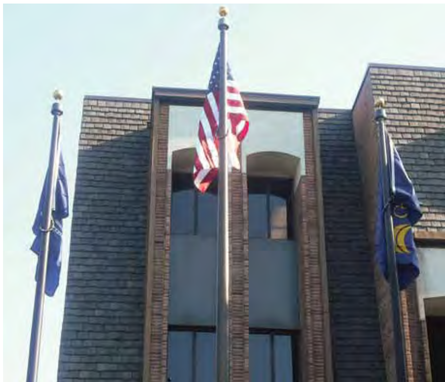
Sneden Hall represents the initial phase of the college’s long-term plan and provides room for 86 class sections and 750 students on a Monday through Thursday daytime schedule.
